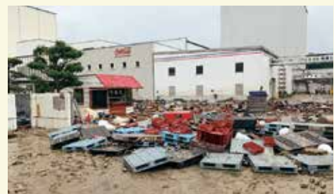
Hongo Plant after the flooding
