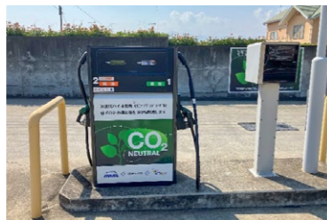
Renewable diesel-compatible fuel pump
